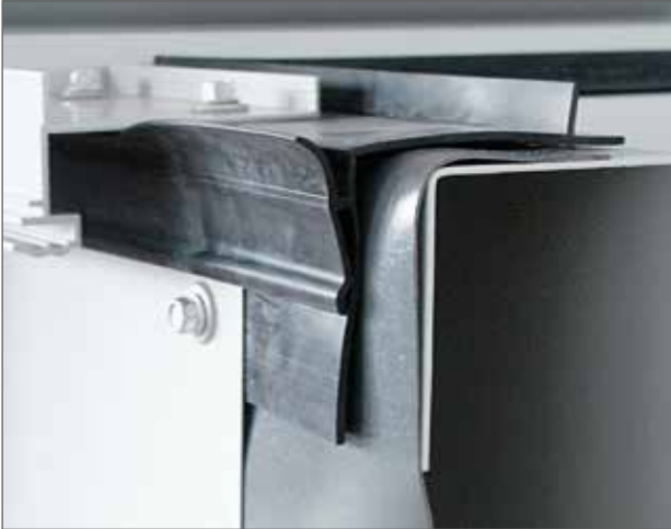
Frame safety connection for classic arcade rooflight
